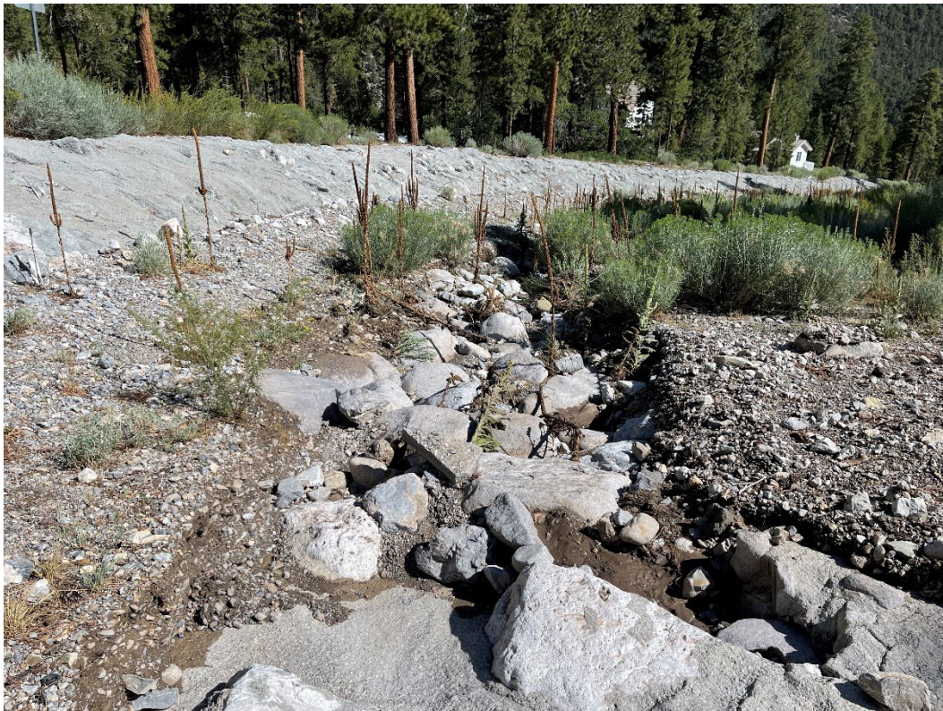
Figure 6 - Runoff entered diversion channel
