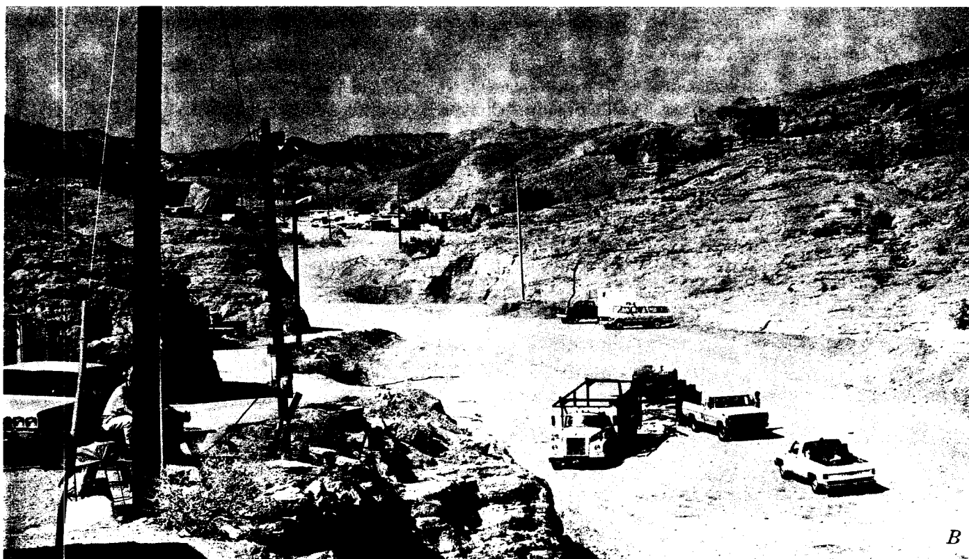
FIGURE 7.—Mouth of Eldorado Canyon. A , On September 14, 1974, probably during the late recession of flooding (photograph by Kenneth E. Beales, Las Vegas, Nevada). B , On October 1 during excavation of flood sediment deposits.
