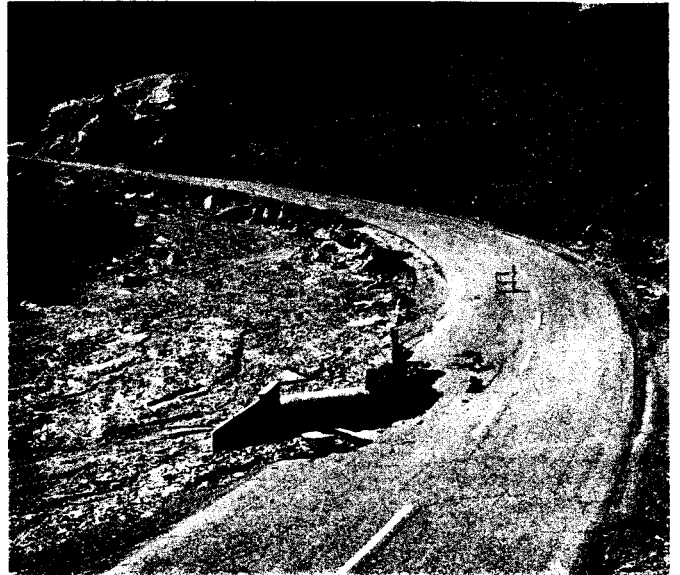
FIGURE 27.—Highway damage in Techatticup Wash caused mainly by lateral channel scour.
