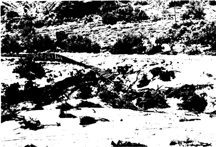
Figure 5. Railroad damage in Moapa Valley.
