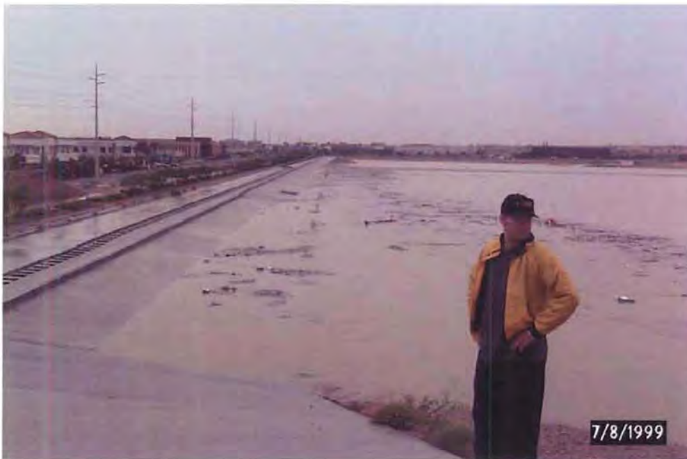
Figure 6 – The Gowan Detention Basin came within one foot of capacity, reaching a depth of 22 feet. Photo Courtesy Clark County Regional Flood Control District.
