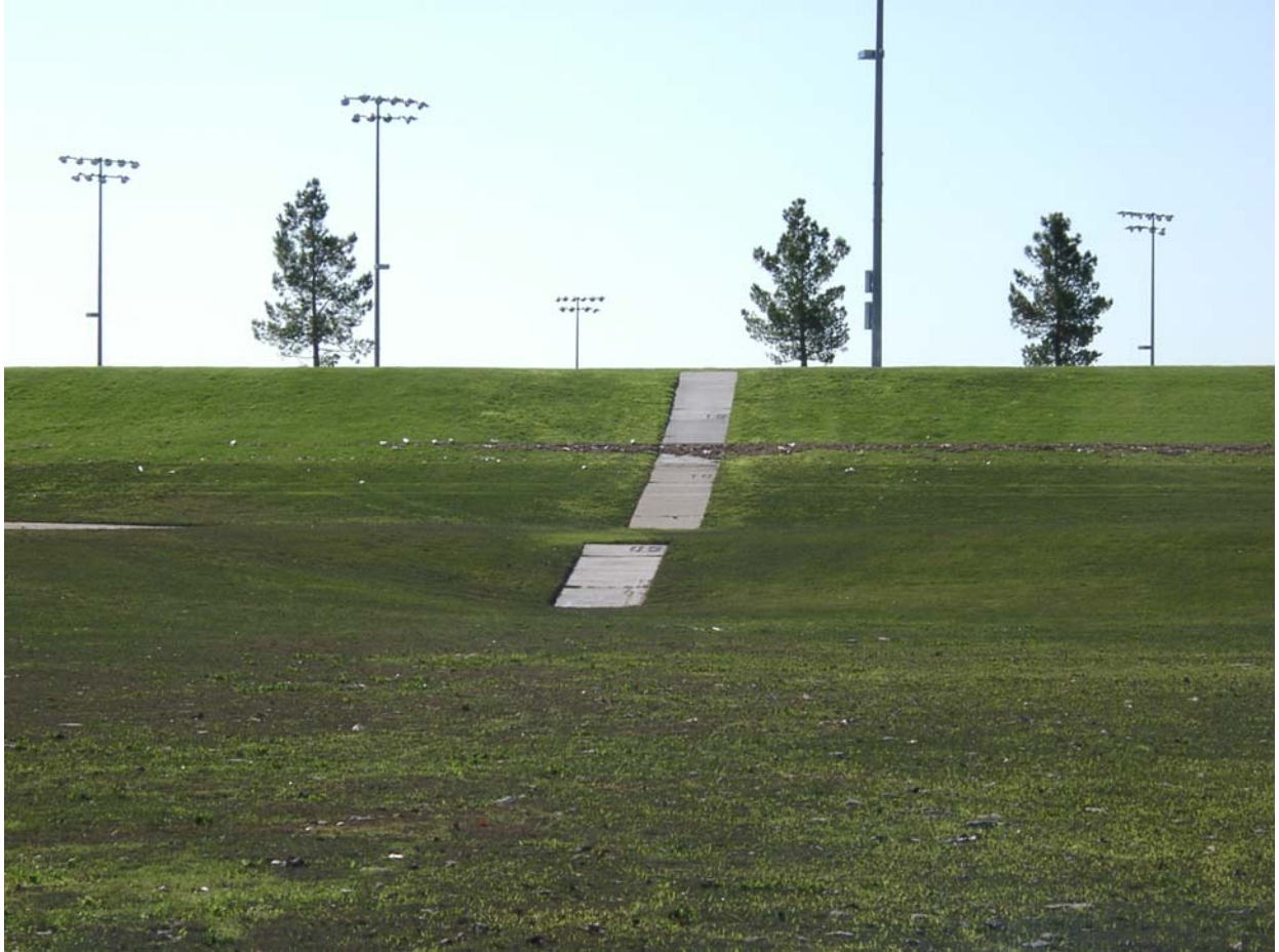
Figure 1. Debris line at The Lakes Detention Basin indicating high water level of approximately 12.3 feet.
