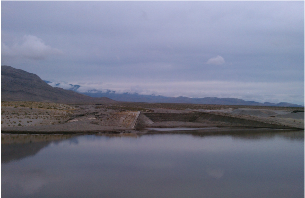
Figure 5. Kyle Canyon Detention Basin (August 26, 2013)
