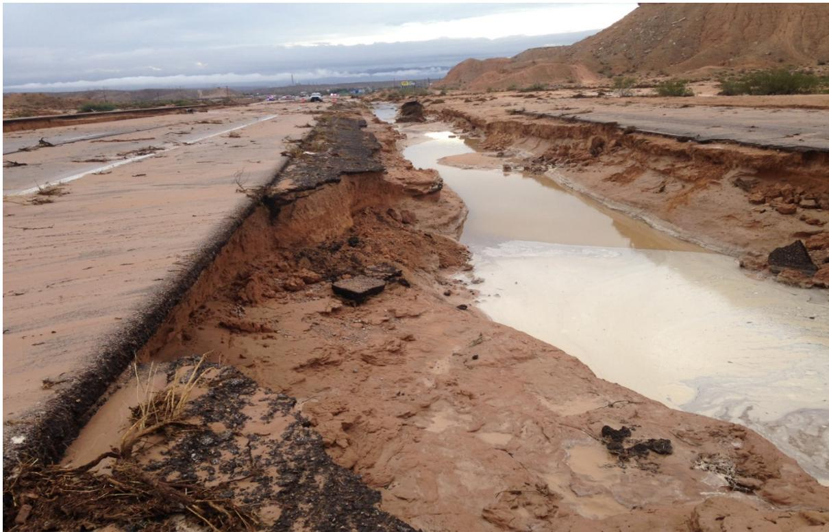
**Figure 6. Damage to I-15 near mile marker 92, September 8, 2014**
