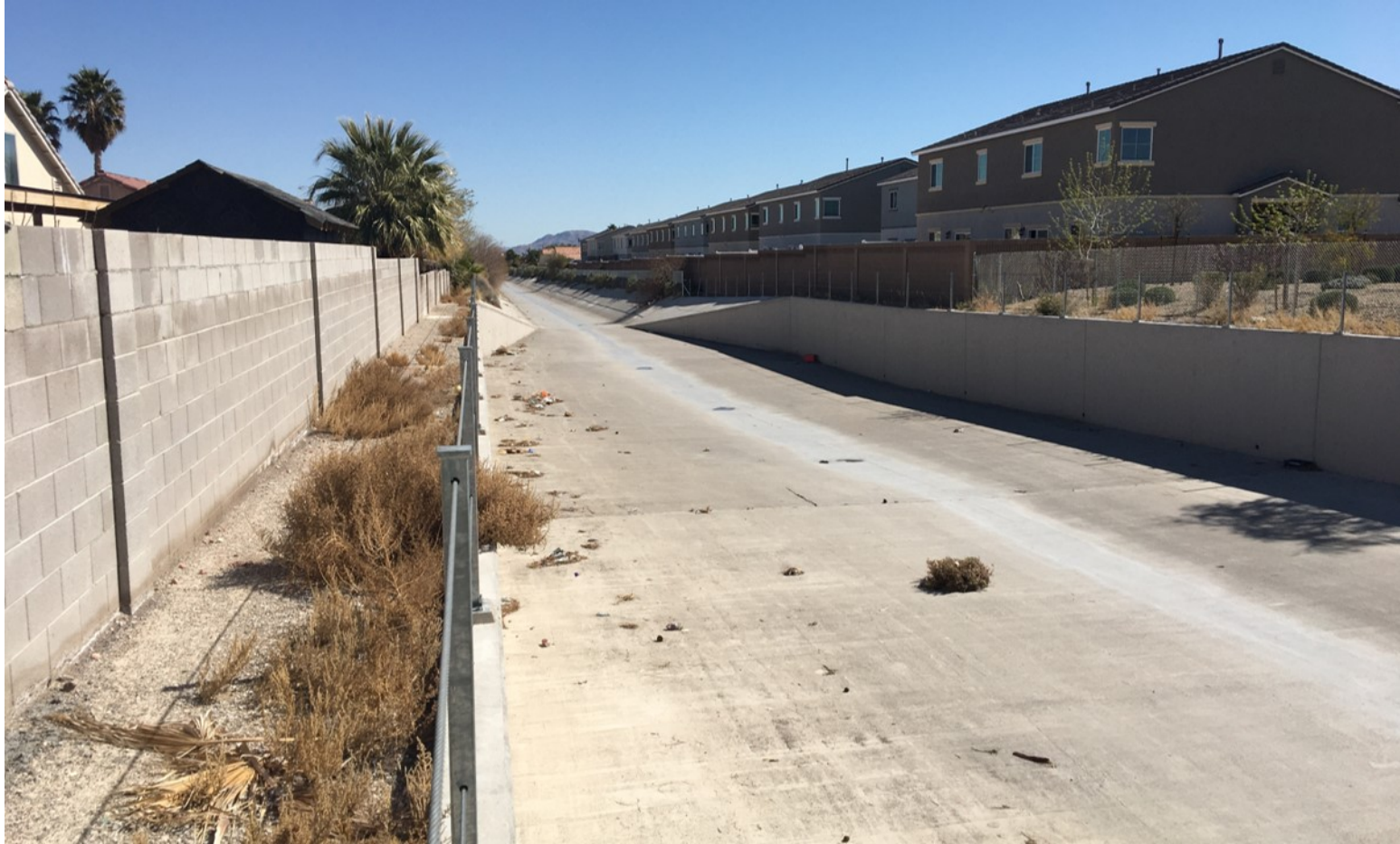
Looking East Along Existing Channel (Red Coach Alignment)
