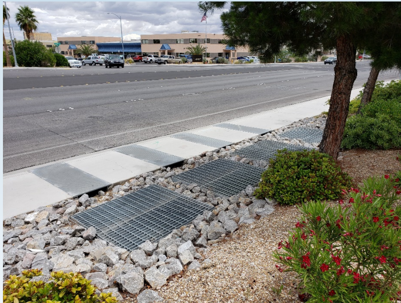
Upstream Bubbler Structure
